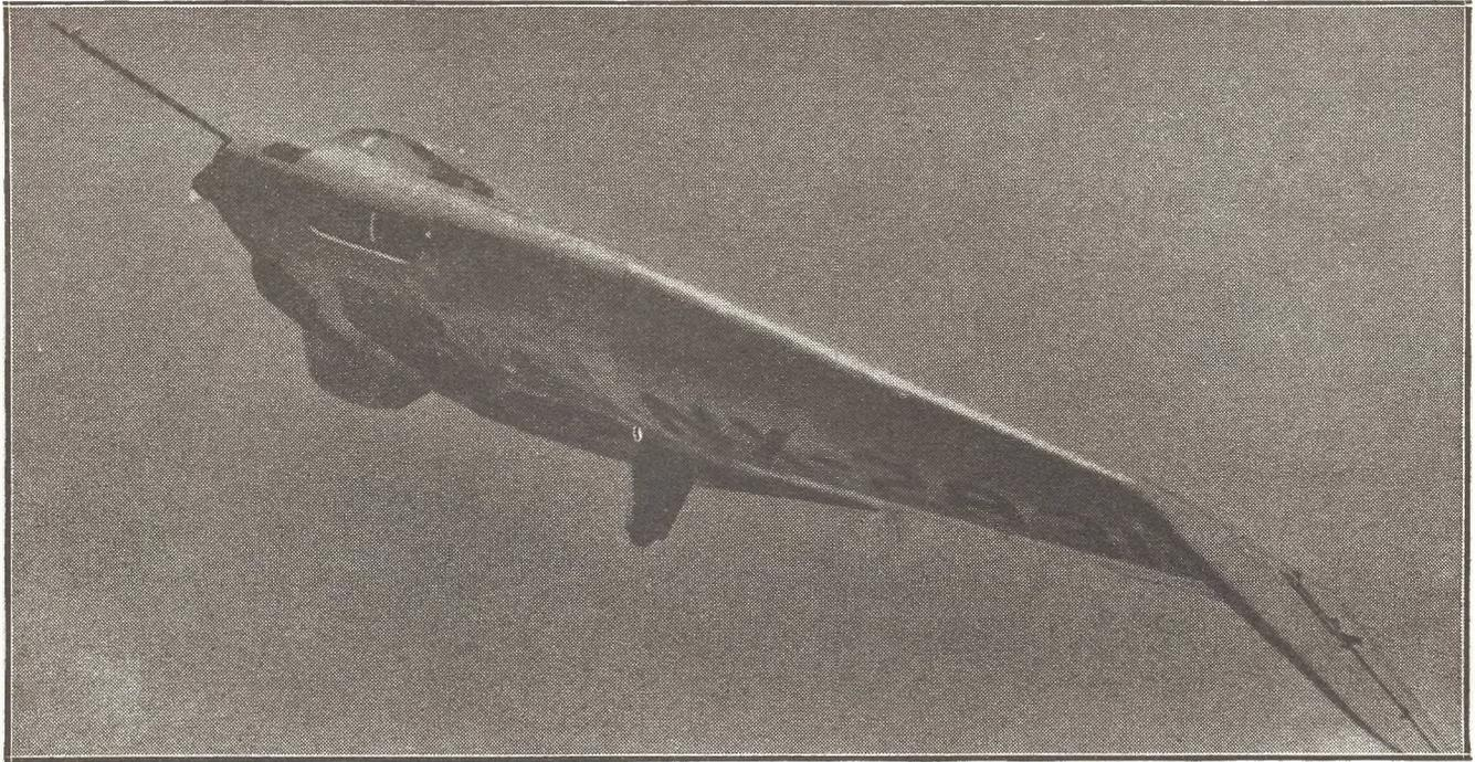
Except for its propeller shaft housings, every square inch of the plane's body increases the lift of the wing. Two 120-h.p. Franklin engines drive three-bladed pusher airscrews.
