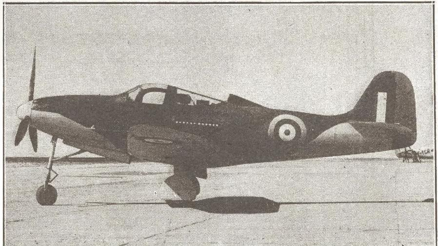
In British service, the Bell P-39 type has demonstrated it is a match for the Spitfire and Messerschmitt up to 16,000 feet.
