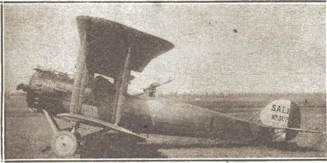
Another famous French observation machine was this two-place job, identified by the markings as being made and powered by Salmson.
