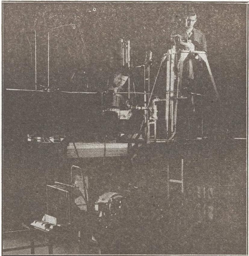
**THIS STRANGE-LOOKING** arrangement of tubes is really the complete fuel system of a modern fighting airplane, brought out into the open where it can be studied under test conditions. The picture shows engineers of Vultee Aircraft subjecting the fuel system to wide-
