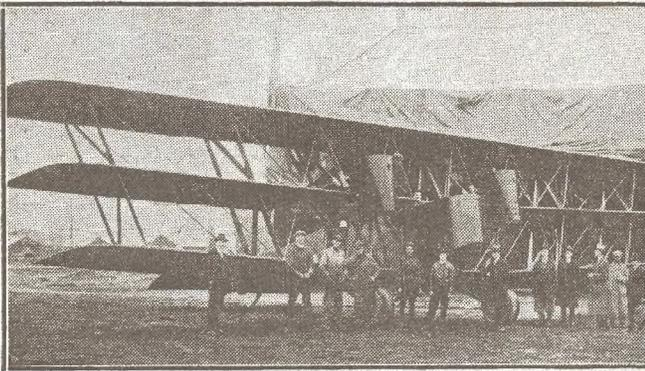
Giant G.A.X. triplane, ten of which were built by Boeing in 1921. Heavily armored, the machines were designed by Army Air Corps engineers. Liberty motors were used.
